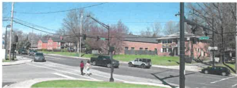
One of two new roundabouts in Kent will be added at the intersection of East Main Street and Horning Road.
